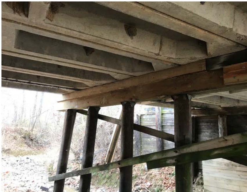
REPLACED TIMBER CAP "A" & "B" AT BENT #1, RT. SIDE
