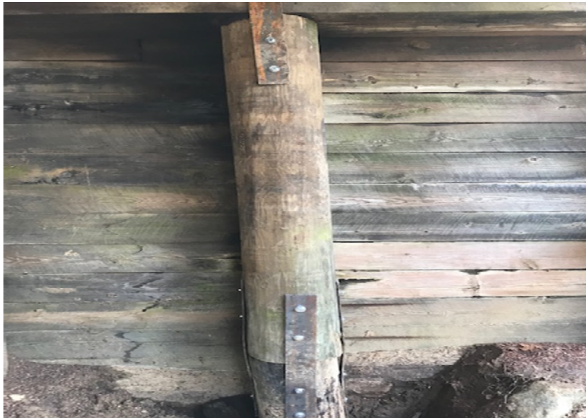
STUBBED PILING "G" AT ABUTMENT #2 7 FT. FROM CAP
