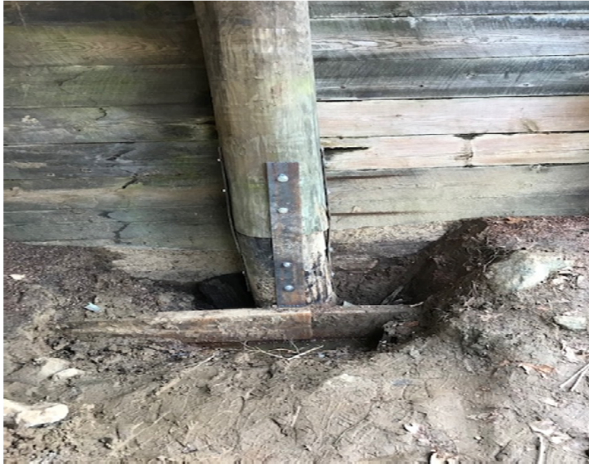
STUBBED PILING "G" AT ABUTMENT #2 7 FT. FROM CAP
